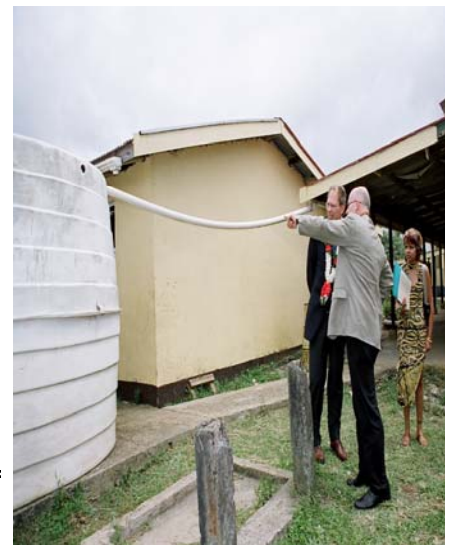
Water Tanks attached to rain water harvesting system on classroom rooftops.
